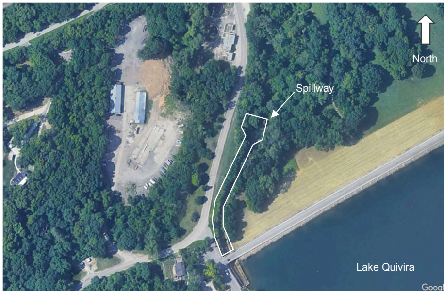
Figure 1. Project Site and Spillway Location
